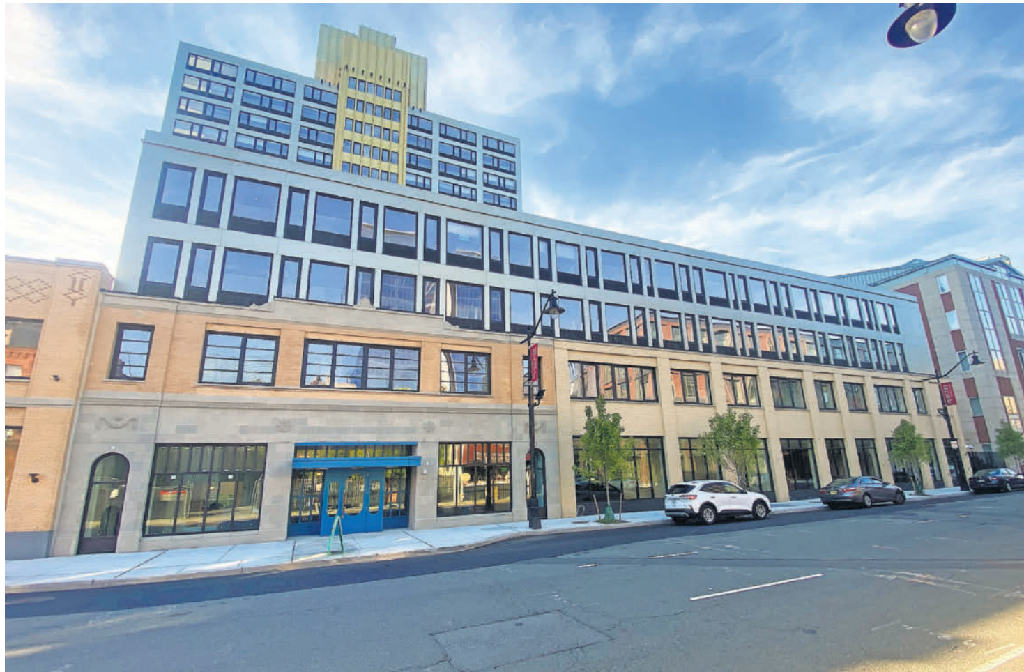
The Newark Urby apartment complex was recently converted from a 12-story parking garage into 250 living spaces. A city ordinance adopted Wednesday limits rent increases to 5% a year in newly constructed buildings. Tyrone Z. McCants, for The Star-Ledger
