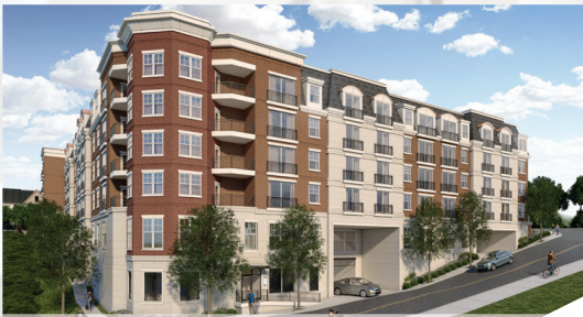
The Residences at 30 Court • Morristown
